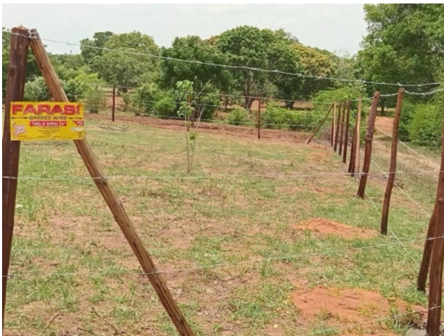
Fig.1: New site secured for building permanent BSF facility and other structures.
